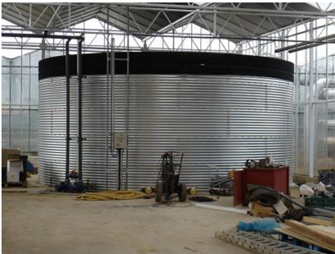
Picture 7: Water storage is required by some businesses to main continuity of water supply.
